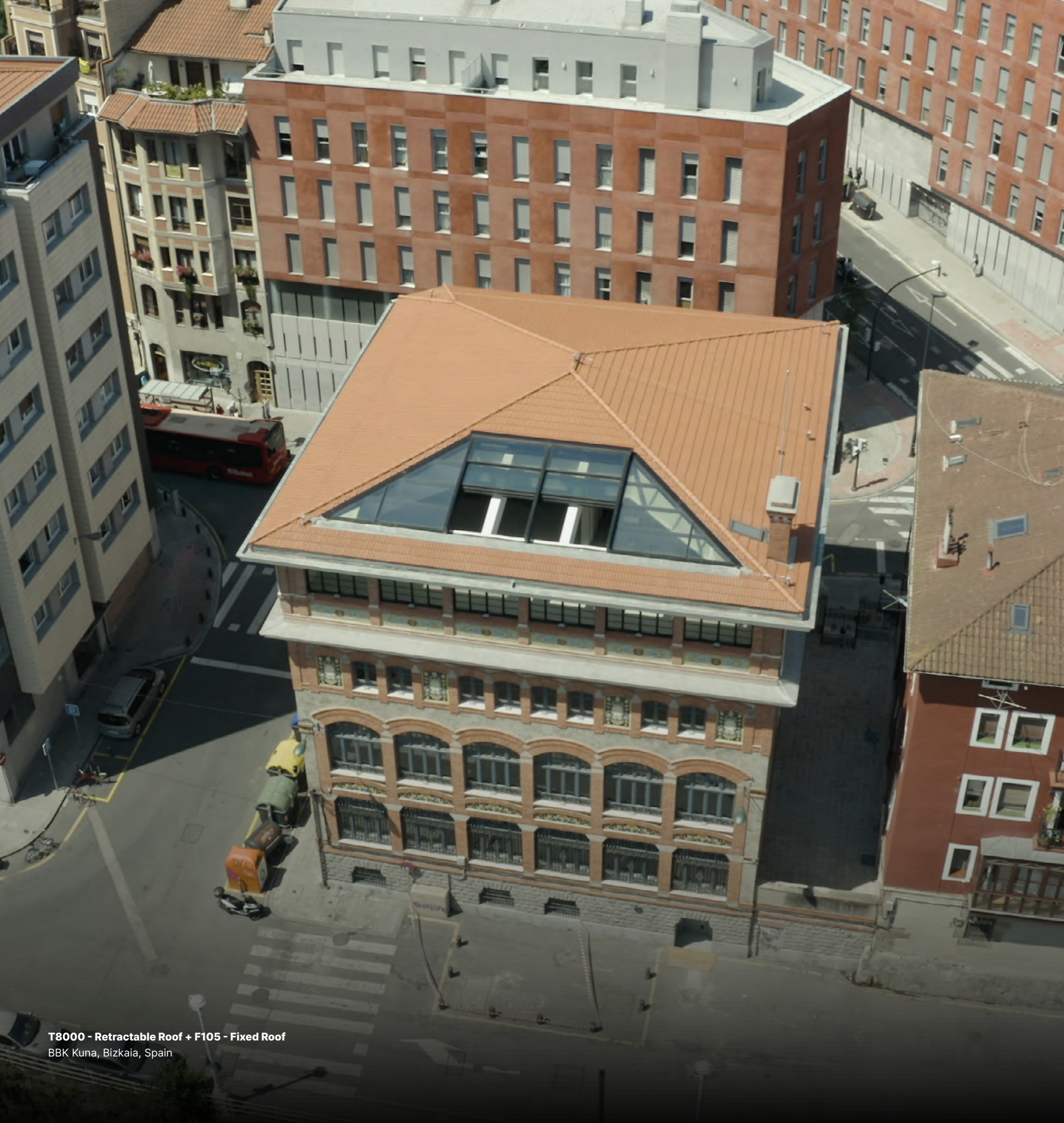
Retractable roof and fixed roof combination - Closed position.
